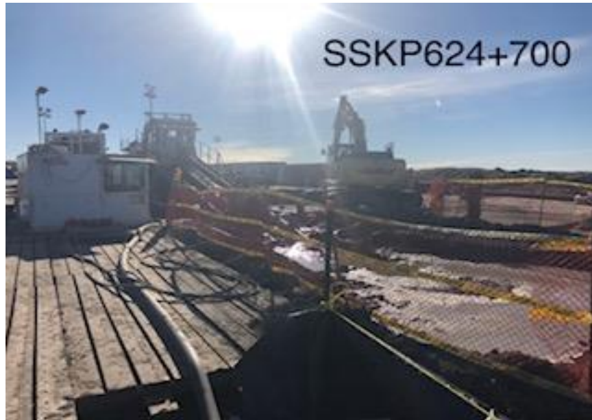
HDD Equipment at entry point
