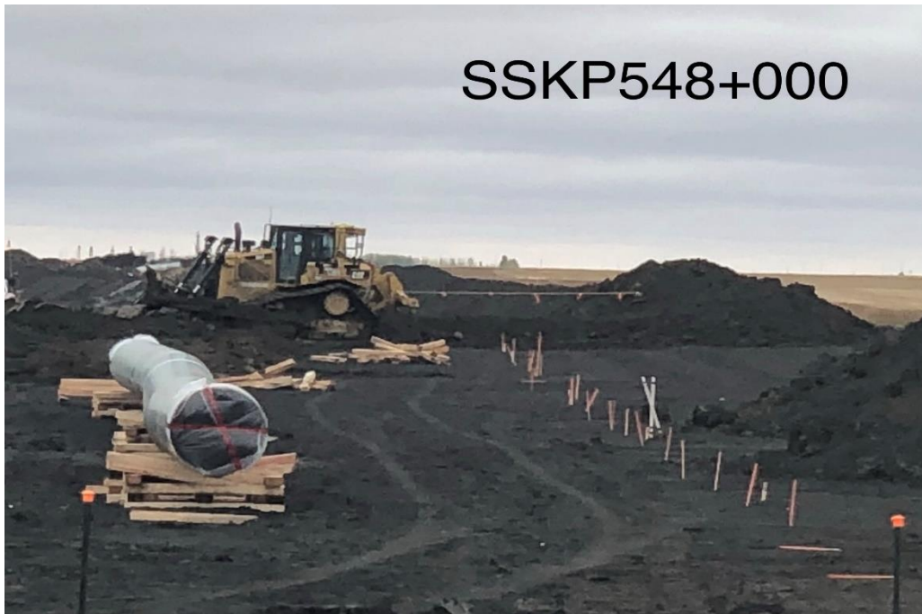
Backfill process
